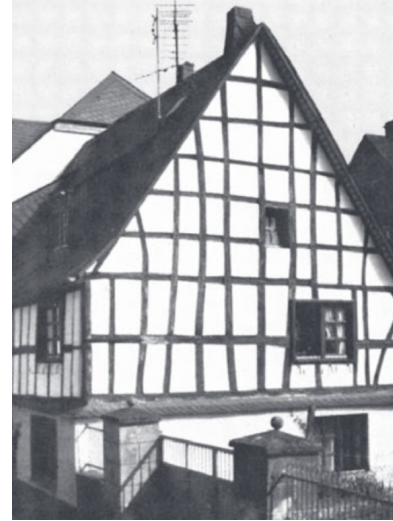
Use of naturally bend timber elements Grossmann 2004
