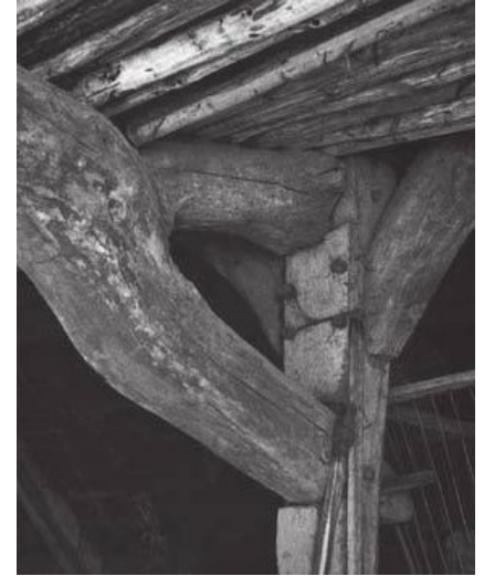
Branch as structural element Kirk, 1994
